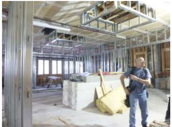
This photo shows framing for two skylights above the open office space in the Chancellors office.
