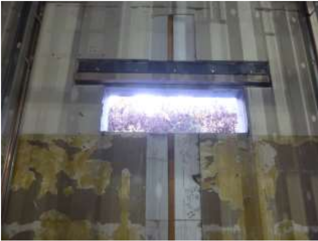
Lower level: One of three openings at the concrete wall that faces the pedestrian path, allowing north light into the ground floor.
