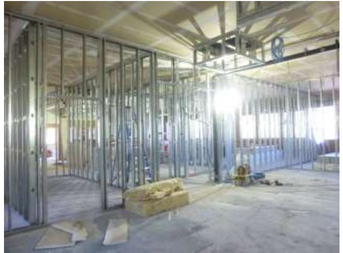
Upper right shows framing for one of four skylights at the upper level.
