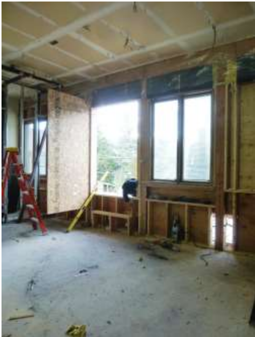
This photo illustrates the height of the new window openings compared to the existing window height.
