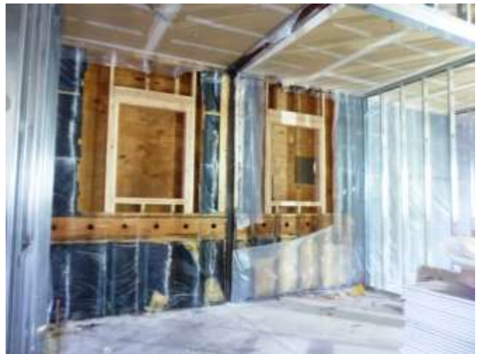
Two new windows are being added at the southwest (back, transverse) wall which opens into the open office space.
